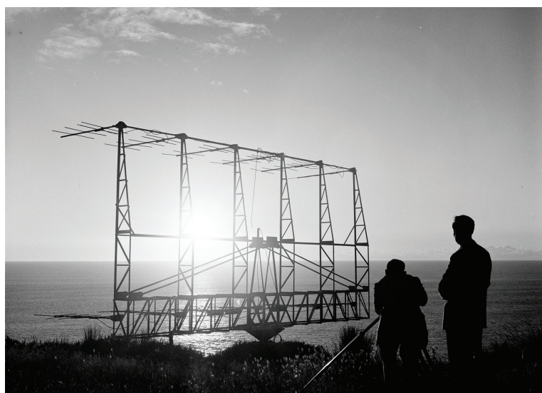
In the early years of radio astronomy, arrays such as this were mounted on the cliff-top at Dover Heights in Sydney's eastern suburbs. This photo was taken in 1955.
