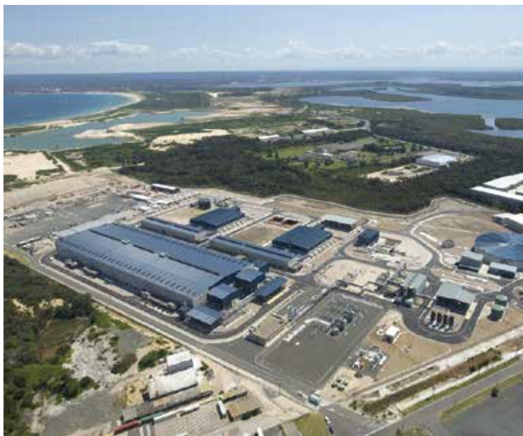
Pentair supplied essential technology for the $1.86 billion Sydney Desalination Project completed in 2010 and designed to provide an additional 15% capacity to Sydney’s supply network. Pentair’s CodeLine membrane housings are used in many of the world’s major desalination projects. Desalination works by treating seawater through reverse osmosis. As the water is pushed through the CodeLine membranes, salt and other impurities are removed, producing potable water.
